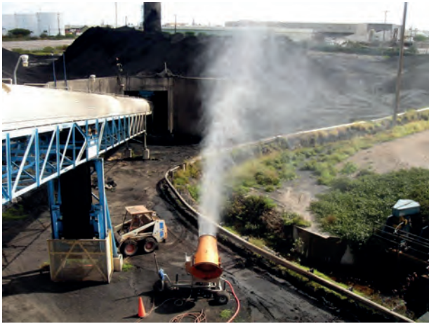
Figure 1. Coal operations need versatile and mobile dust control options that allow them to adjust for changing conditions.
