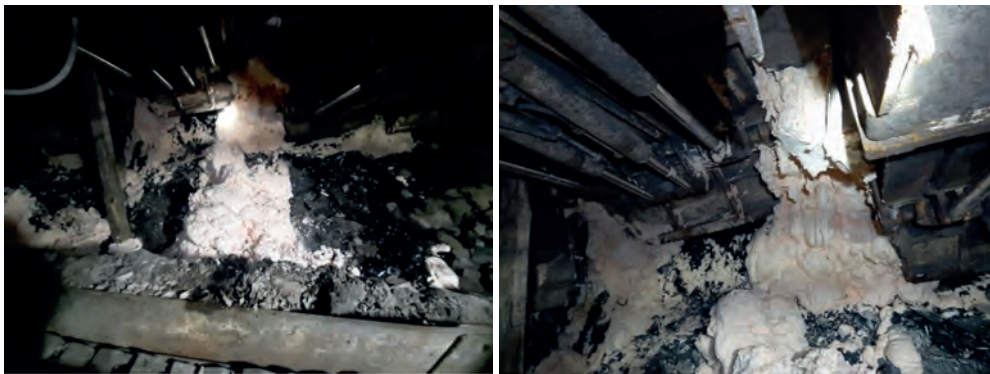
Figure 2. Cavity filling with expansive resin Rocsil Foam.
