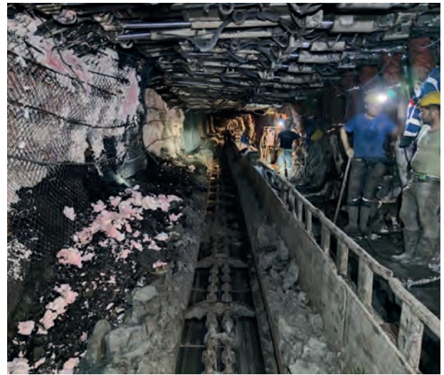
Figure 3. Longwall recovery after foam filling.
