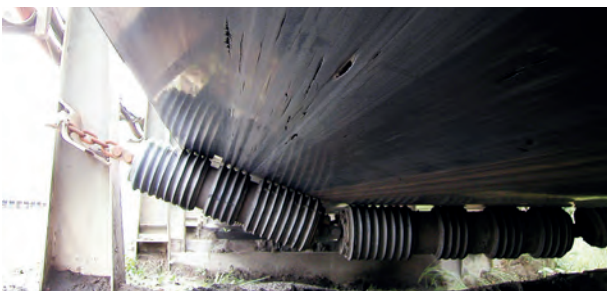
Figure 3. Cover damage that allows moisture to reach the cables.
